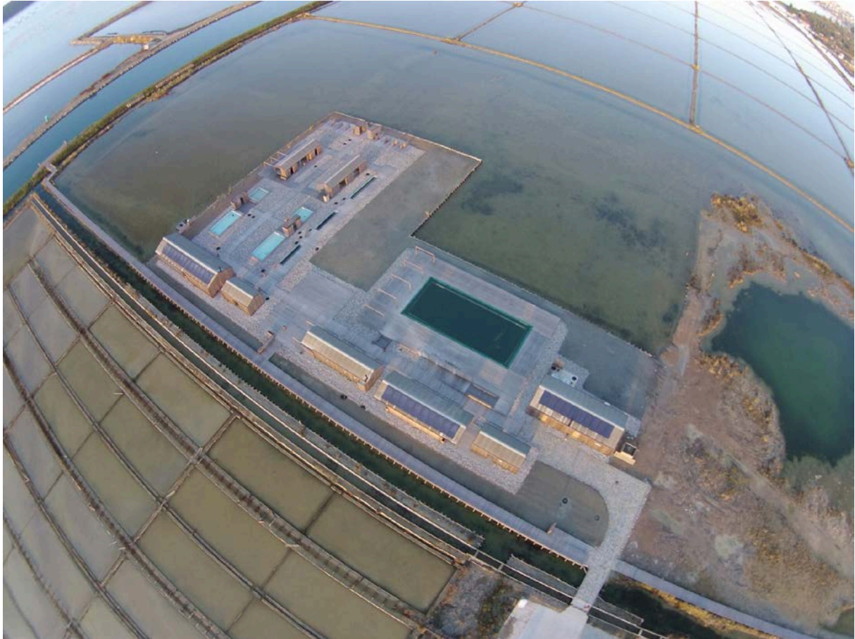
Figure 2: Aerial view of the Thalasso Spa Lepa Vida complex (photo by: I. Škornik, KPSS)
