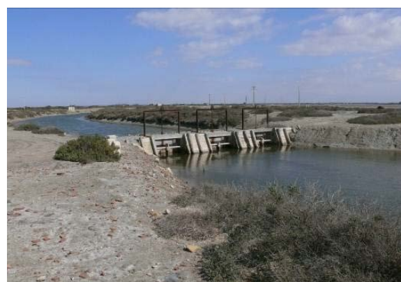
Old Hydraulic sluice system
