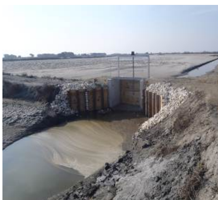
Restored hydraulic sluice system
