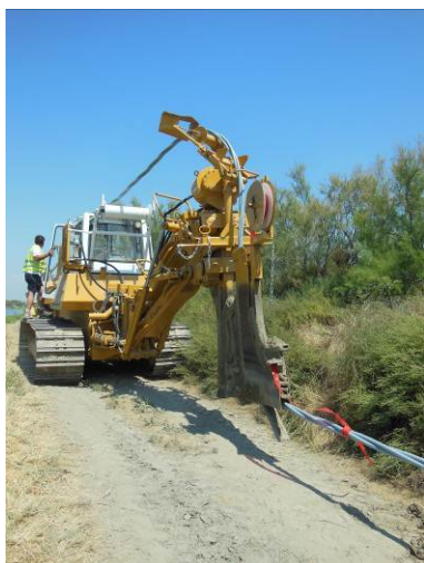
Machine used to bury electrical cables
