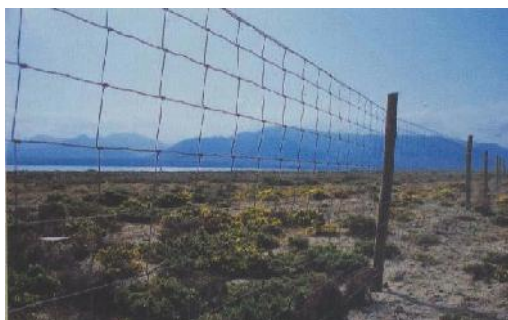
Figure 4: 11km of 1.4m-high fencing
