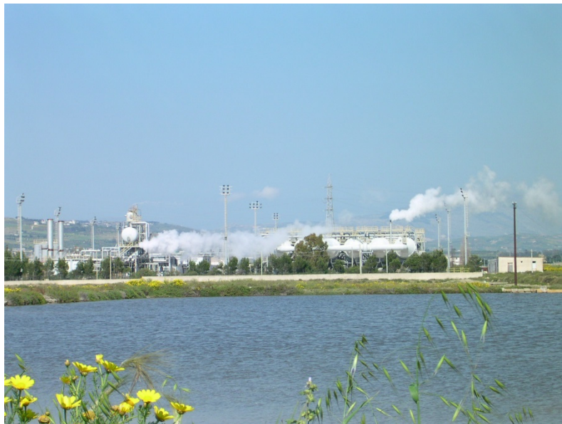
Fig. 1 View of a basin of "Mariastella" saltworks with the MED-TVC plant in the background.
