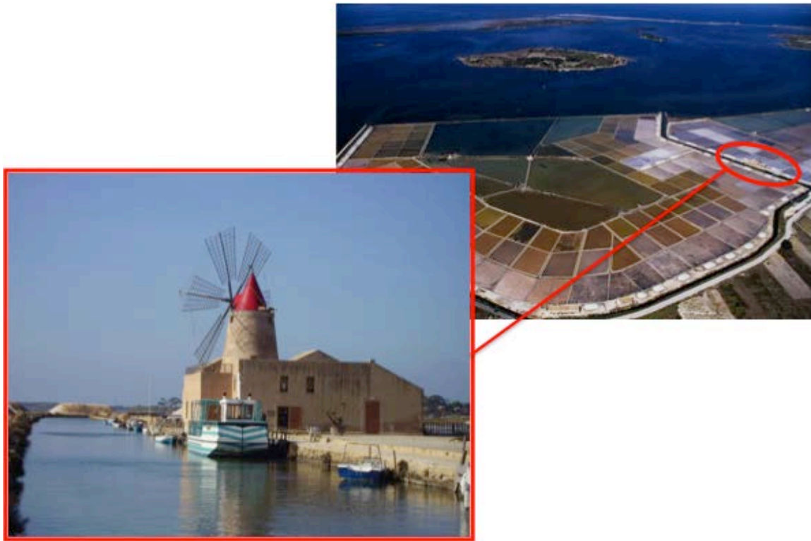
Fig. 16. The installation site of the REAPower prototype: the windmill at the Ettore e Inversa saltworks, Marsala (TP), Italy.
