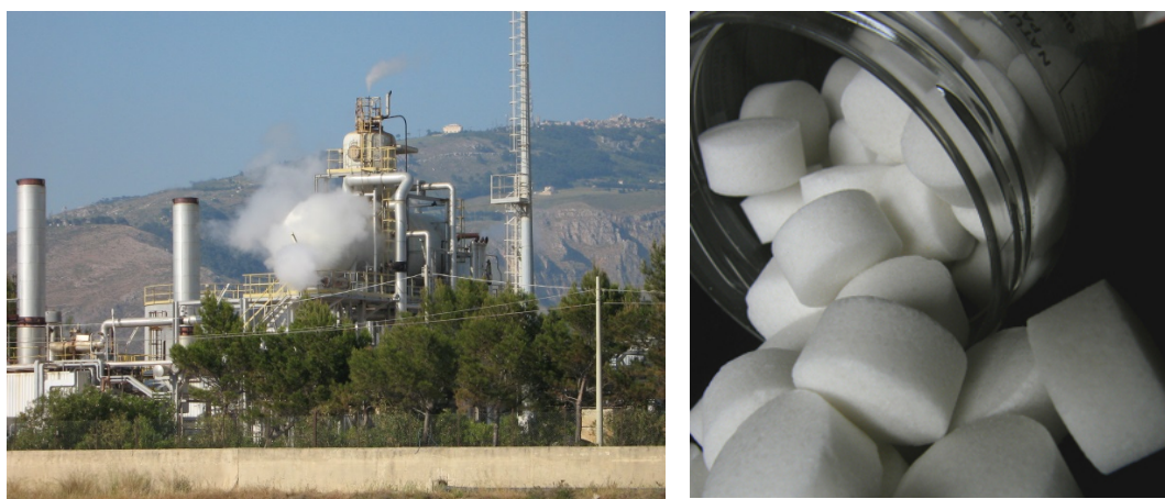
Figure 6 – Desalination plant of Trapani (left) and water-soluble natural integral sea salt tablets (right), ph http://www.flamingosalt.it/ .
